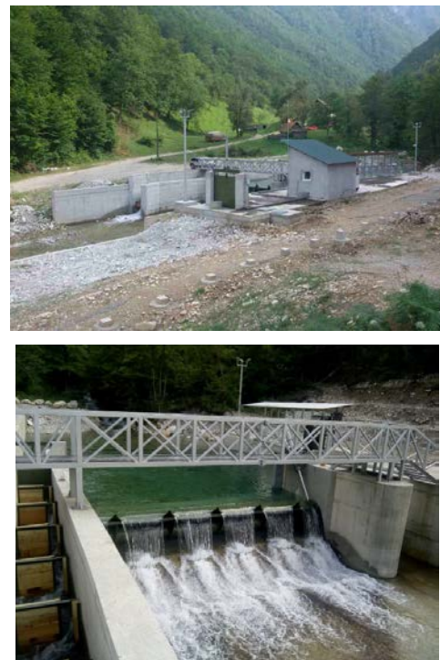
Figure 15. Water intake of the Bistrica Majstorovina SHPP
