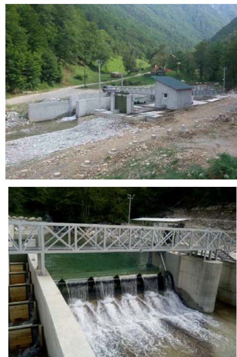
Figure 15. Water intake of the Bistrica Majstorovina SHPP
