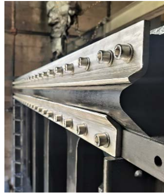
Figure 7. Gate top seal after refurbishment
