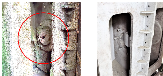
Figure 5. Before (Left) and after (Right) sand blasting
