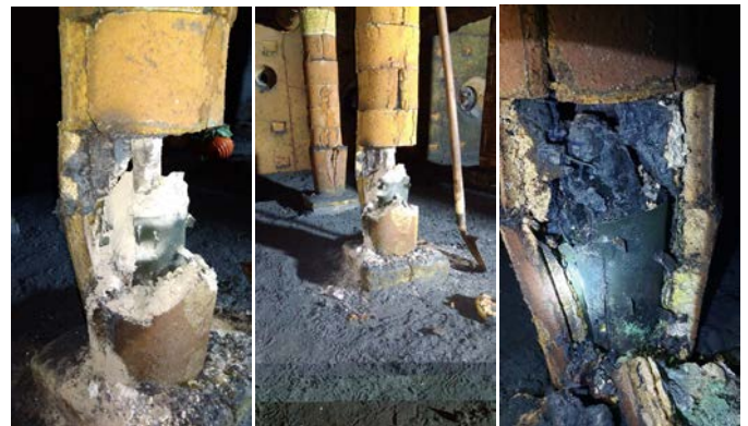
Figure 3. Damages occurred at the vertical girders
